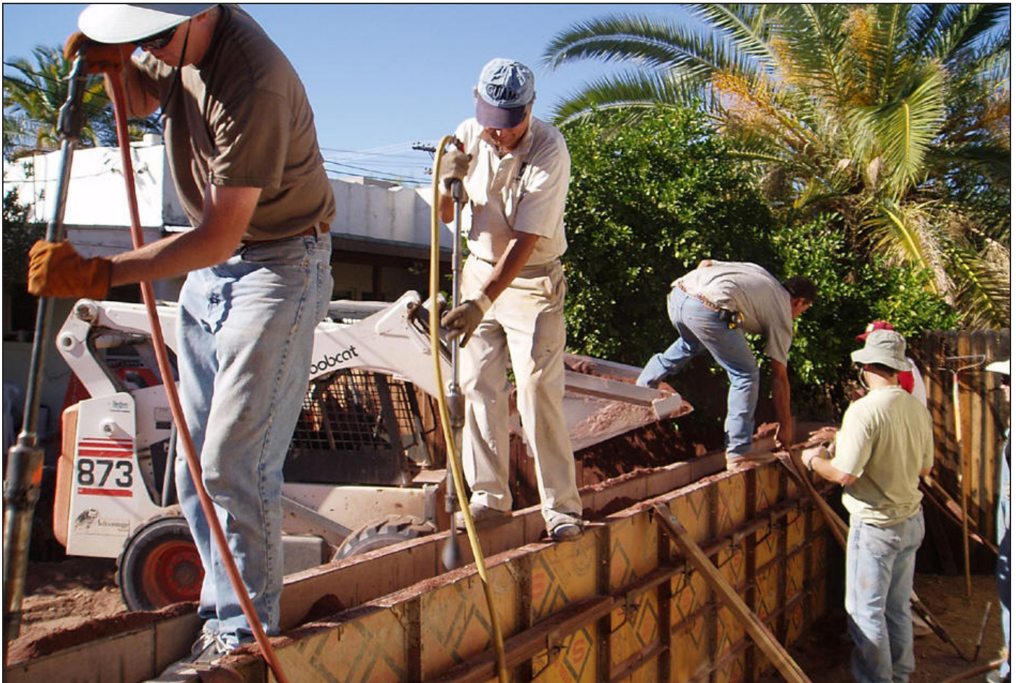
Soledad Canyon's work crew use rammed earth techniques to build their modern homes.
