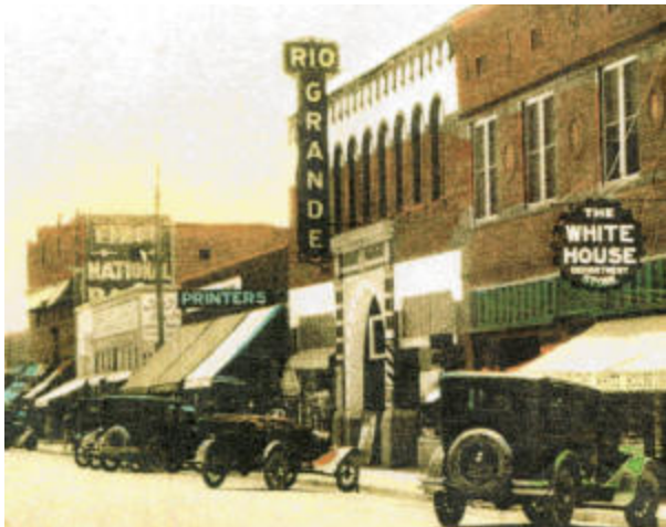
A historic shot shows the Rio Grande Theatre in its early days. The theater first opened in 1926 and has weathered earthquakes, a fire and hard economic
